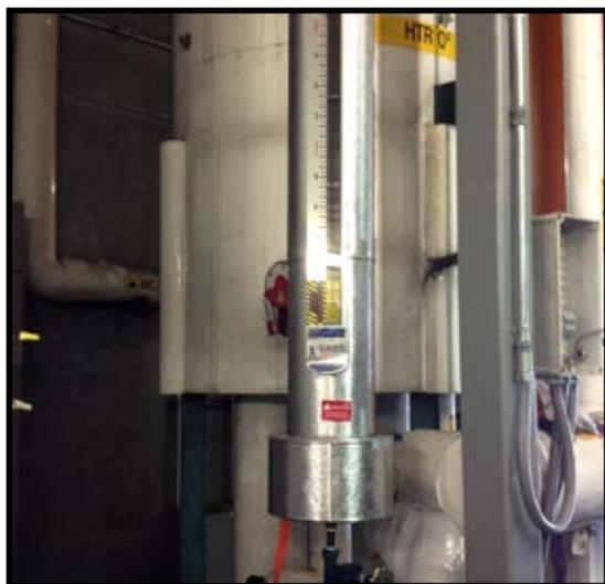
MLI in ammonia service with cryogenic insulation
